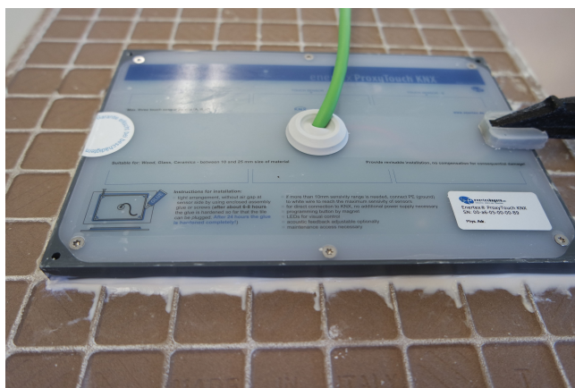
Figure 5: Spreading the mounting adhesive
